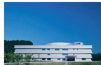
RD1 headquarters building
