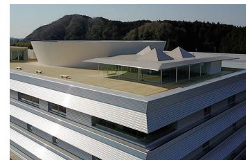
Building exterior showing Sigma environmental control panels
