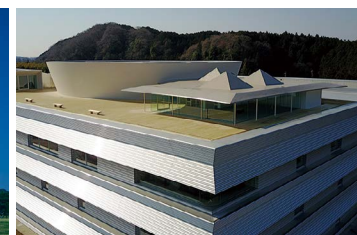
Building exterior showing Sigma environmental control panels
