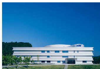
RD1 headquarters building
