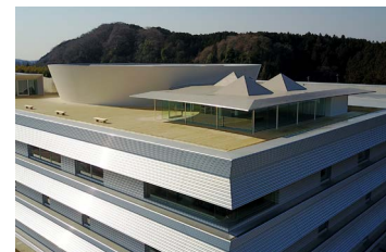
Building exterior showing Sigma environmental control panels
